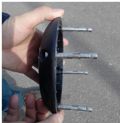
Figure 9 install 4 expansion screws
